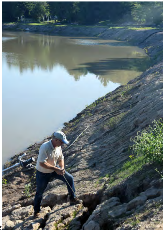
Area 2 Engineer Todd Zielinski surveys a portion of the former lake bottom of Sanford Lake.
